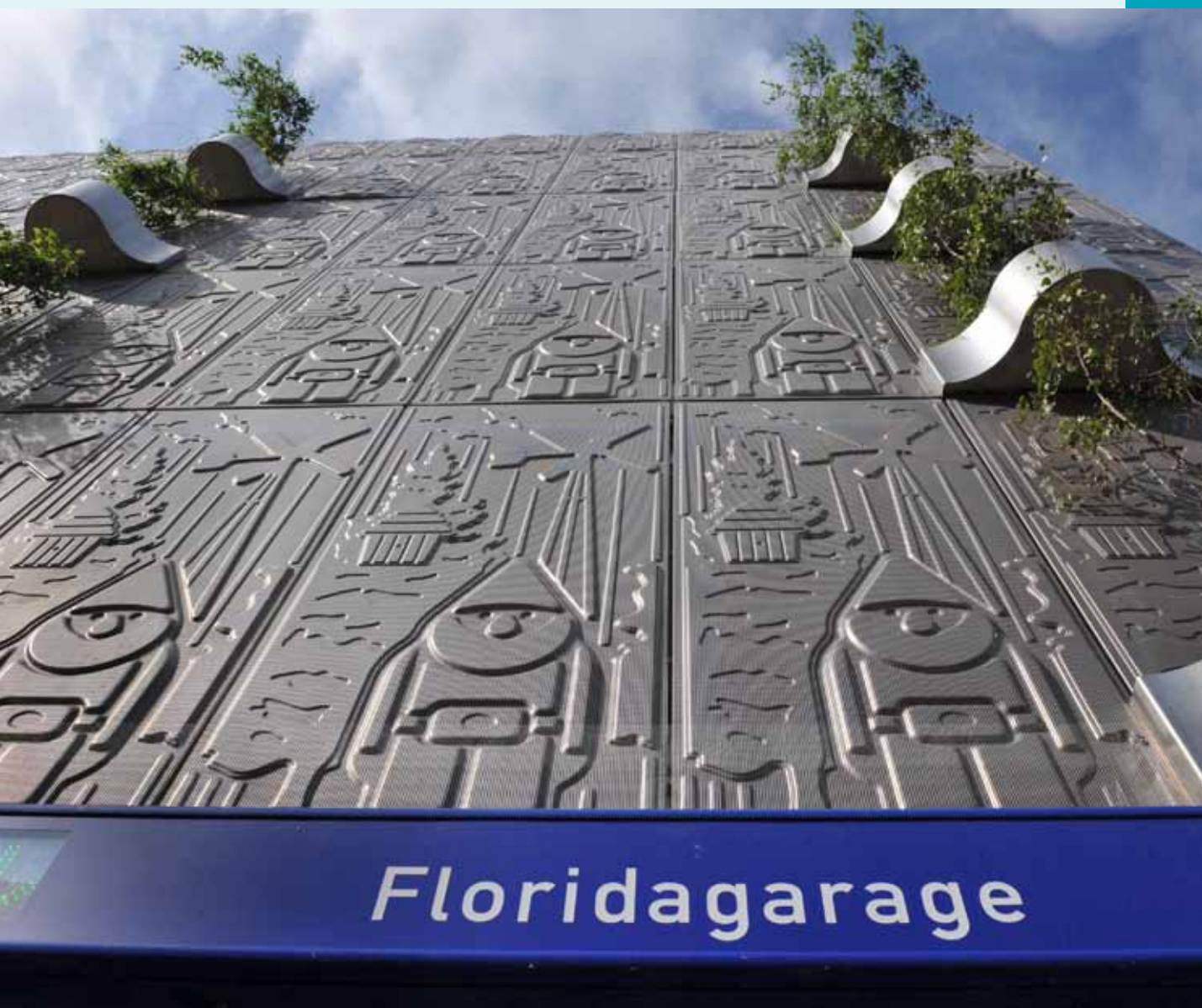
Floridagarage Almere Buiten, growing green building.
